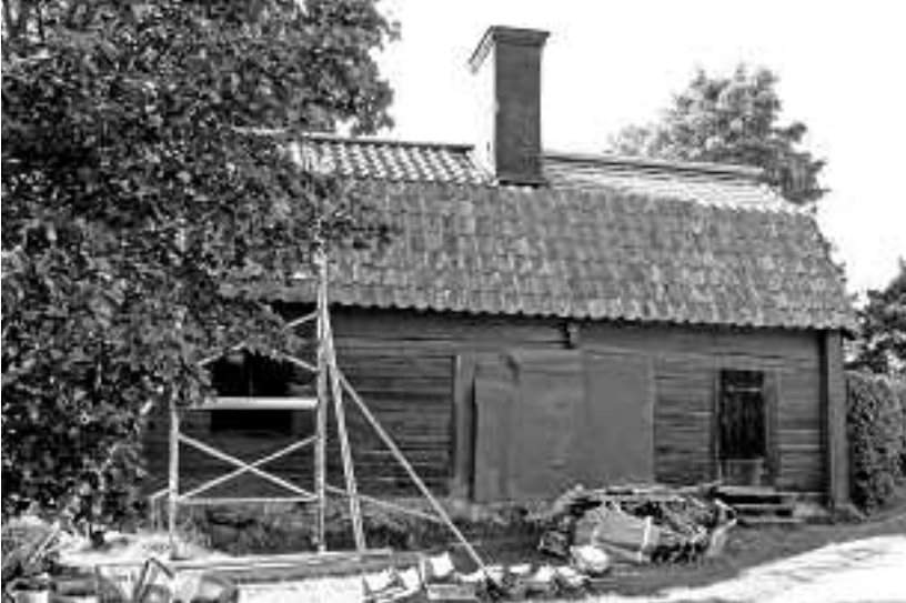
Bagarstugan under reparationen
